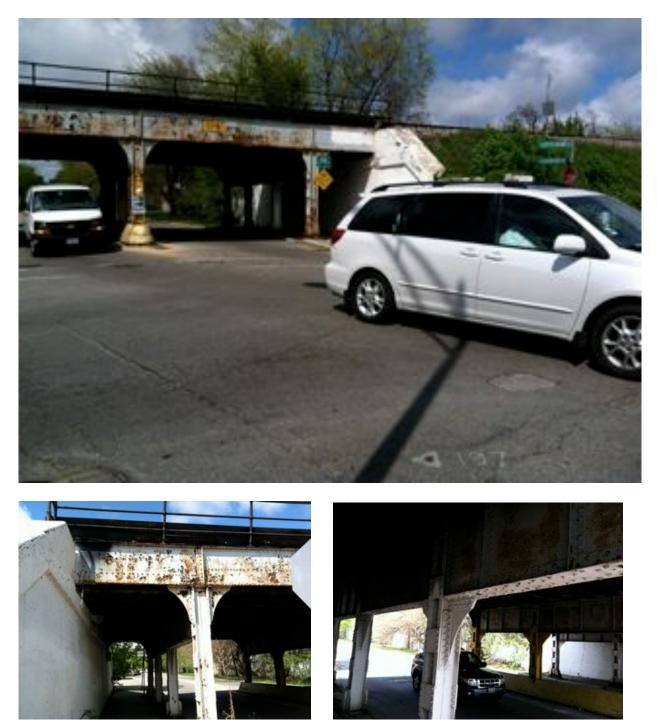
Above we see rivet and column detail. It is a highly riveted structure (that's why it has lasted). Rivets move and allow a bit of structural flex. Weldments would have been more solid, stressed, cracked and have a greater propensity for failure. Rivets while allowing movement show rust stains and paint distress (flaking, peeling and loss) at locations of movement. Hence, you can visualize how a structure is behaving by examination of its individual components.
