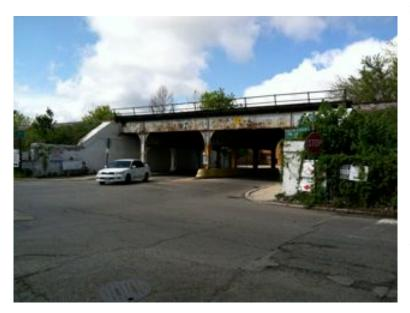
rectangle with 11'-6" painted immediately over the right lane. We now have the vertical elevation. Take any ruler and convert to find feet and inches: I estimate the span to be 36 inches flange to flange across the face. The opening for the left car lane is 14 feet by estimation. You can deduce the others as a challenge.
